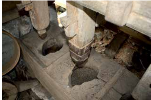
Figure 3. Inside view to stope.
